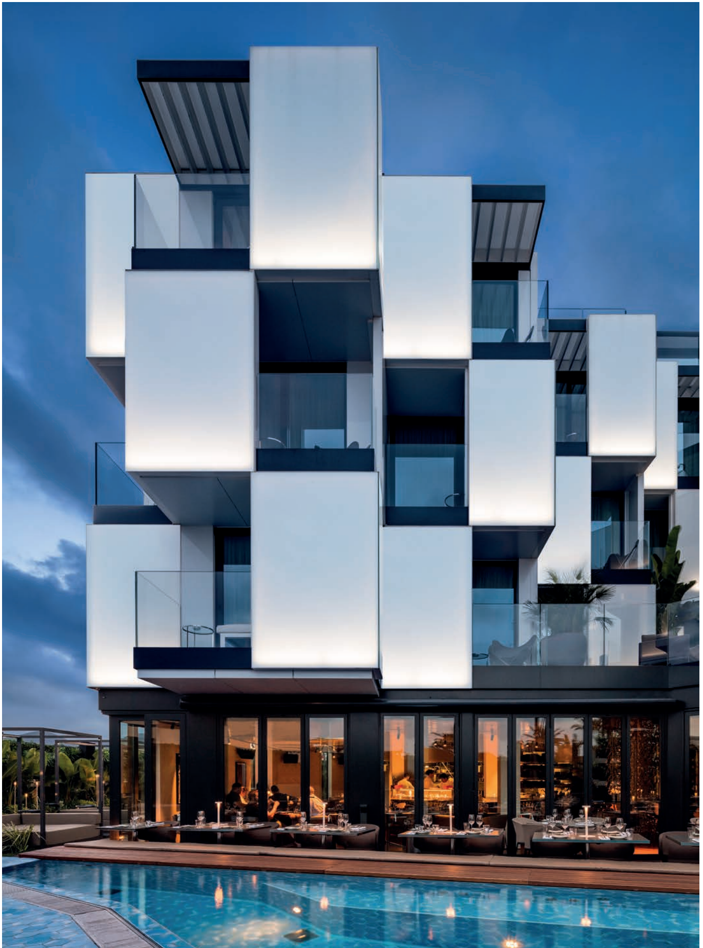
Hotel Sir Joan, Ibiza. Architects: Ribas & Ribas arquitectos. Photography: ©Lluís Casals.
