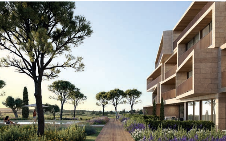
Lumare, currently under construction, explores the light and coastal setting of the Algarve
