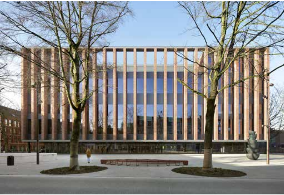
Bruges Meeting & Convention Centre (Brujas). Foto: ©Filip Dujardin
