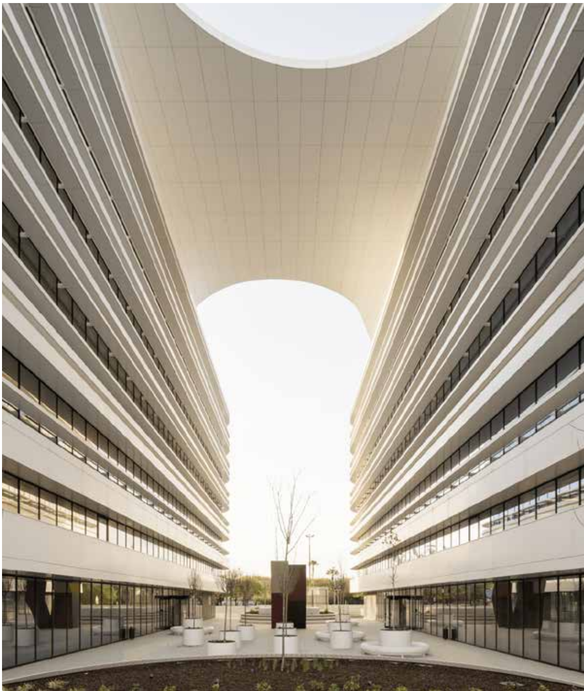
Allo | Alcântara Lisbon Offices. Photo: Luís Nobre Guedes
